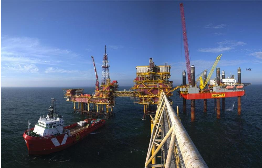
The Seafox 4 currently is contracted by ONEgas and stands alongside the Leman Alpha AC jacket to deliver accommodation and hook-up services.
